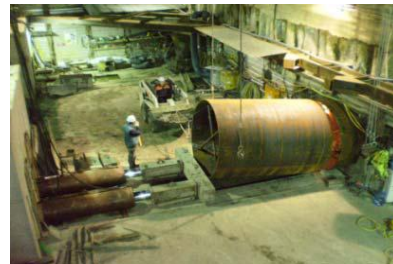
(b) Pressed in steel pipe for metro tunnel
