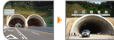
(b) Conversion from twin tunnels to one single tunnel
