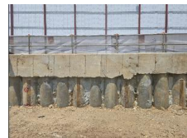
Fig.1.2 Installation of MPG for cut-off wall
