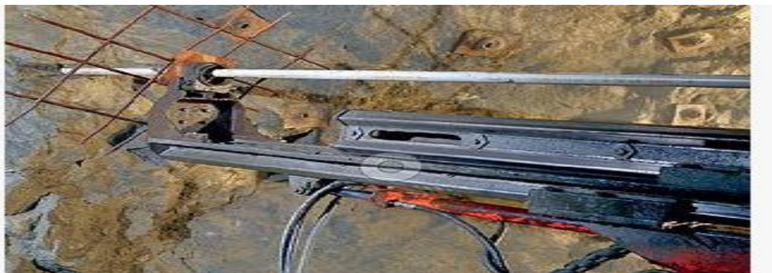
Figure 2 - Installation of the contour reinforcement cage
