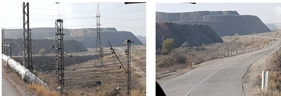
Figure 1 - Ash waste accumulators (photo by the authors)
